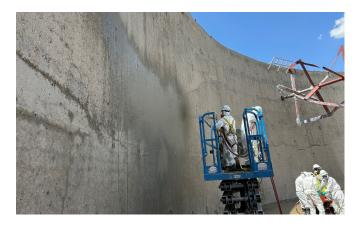
Sunland Construction, the general contractor, self-performed the application across six tanks using Xypex Concentrate (primary waterproofing), Xypex Modified (enhanced protection in high-stress zones), and Xypex Patch'n Plug (for crack repair prior to treatment).
